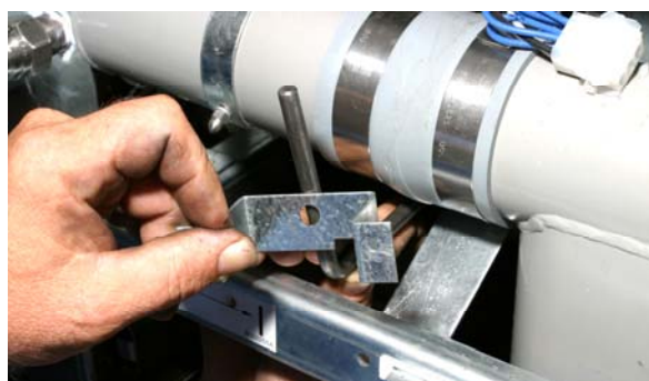
Figure 4: The rod is shown just under the drain manifold. The brace is fastened to the cross brace using existing holes.
