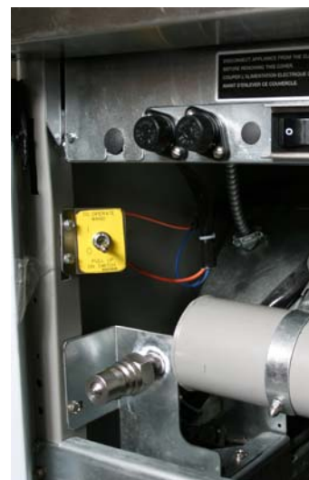
Figure 11: The momentary switch and the front-discharge quick disconnect are visible in the cabinet.
