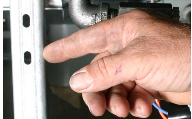
Figure 5: The brace for the U-bolt, which supports the rear discharge plumbing should align with these holes in this vertical brace.
